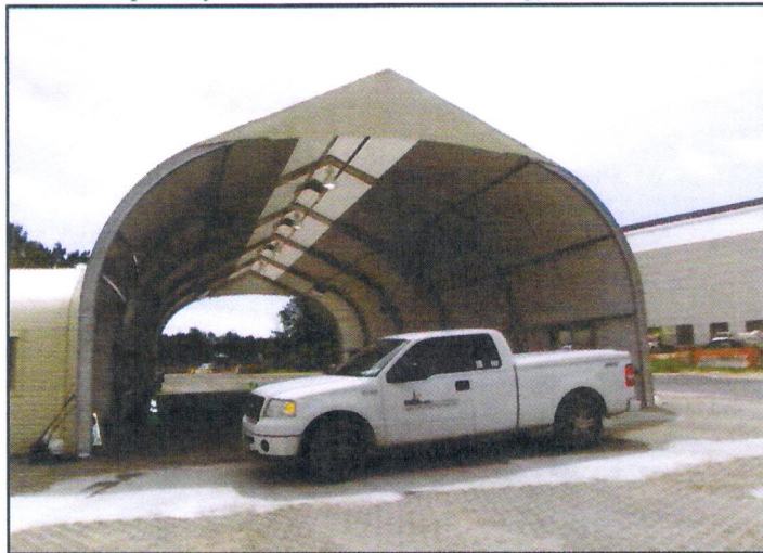
Entrance Canopy is completed at the Joint Base McGuire-Dix-Lakehurst.
